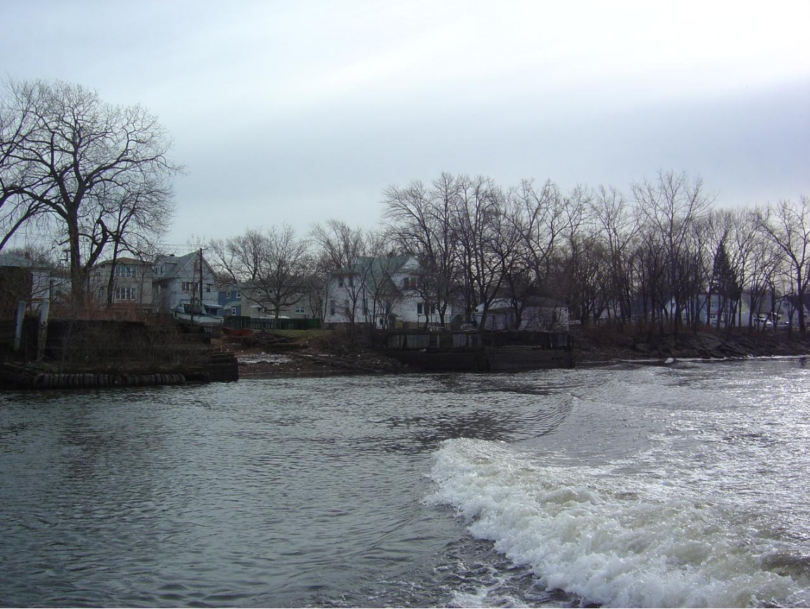
Site 10TMS looking East
